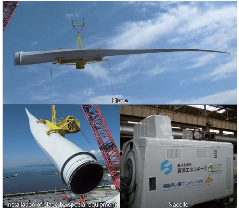
Installation of blade by special equipment
